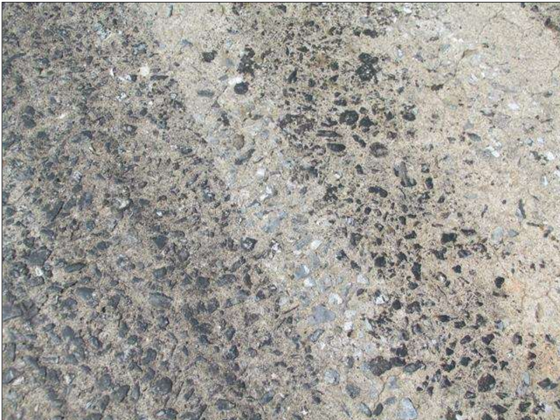
COARSE AGGREGATE EXPOSED THROUGHOUT TOP OF DECK
