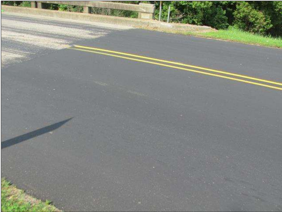
NORTH APPROACH AND SOUTH APPROACH ROADWAYS RESURFACED
