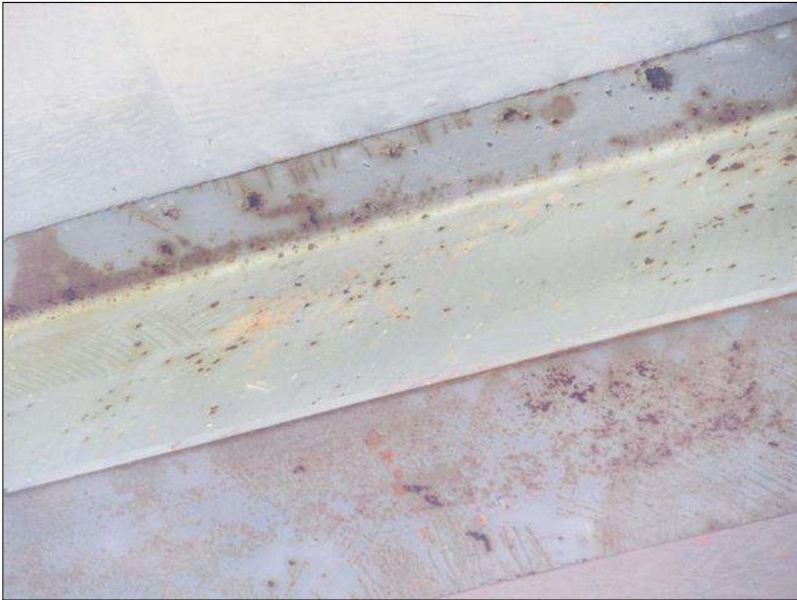
SCATTERED SURFACE CORROSION ON BEAMS
